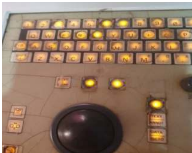
Image 2: Erased knobs and cracks on the control console
